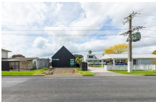
Beachlands – in progress
