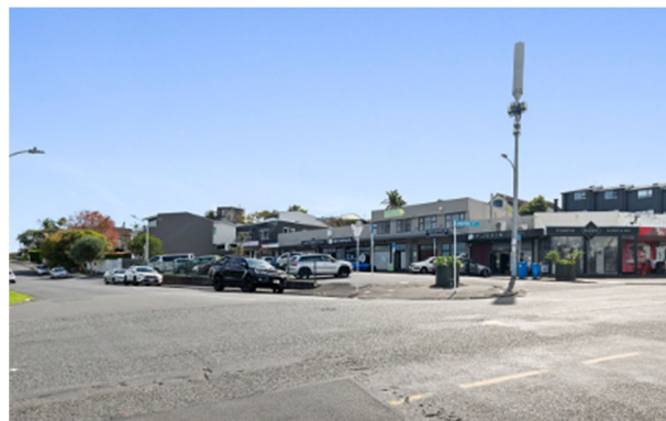
Waimarie Street/Riddell Road, St Heliers (after).
